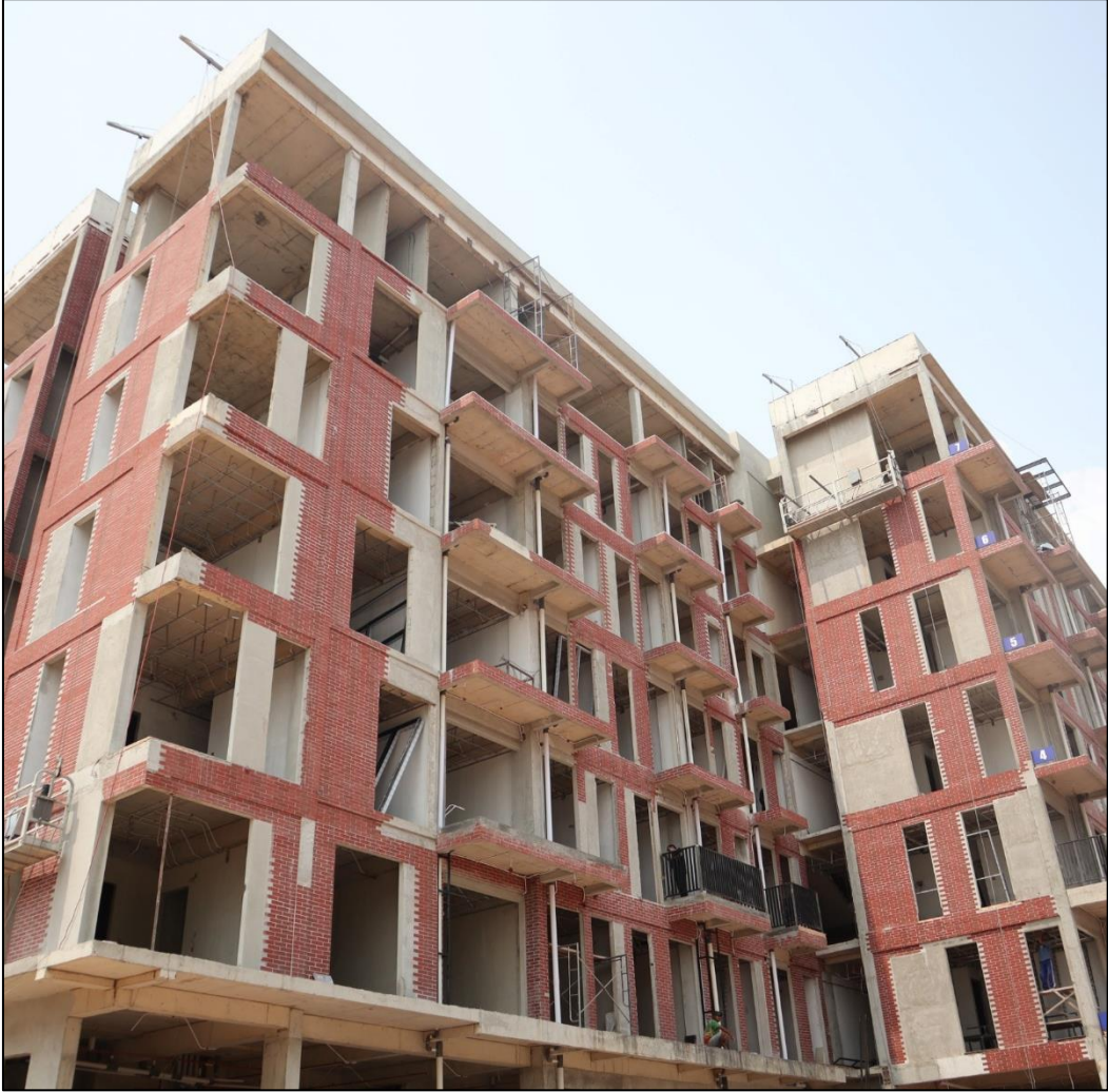
2 MANSORY, PLASTERING WORK (CONDOVILLA)
