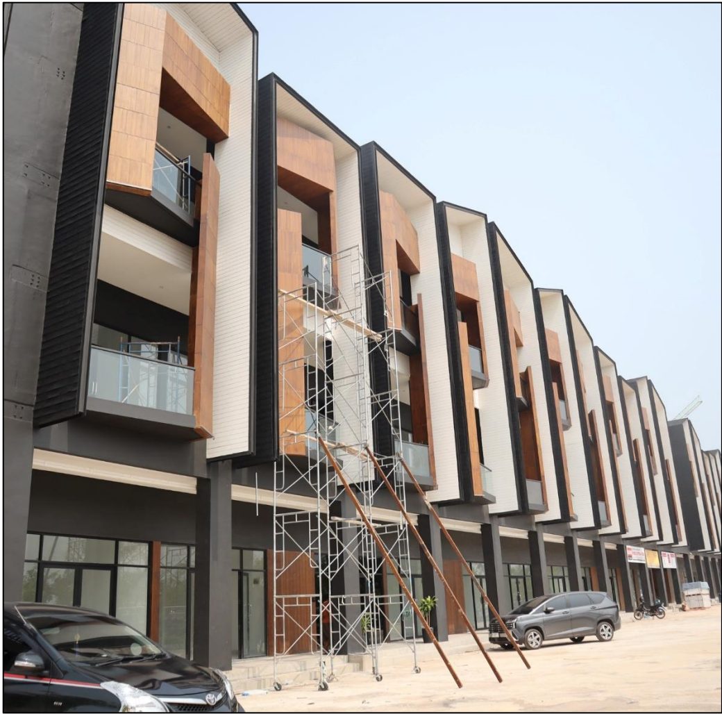
3 CEILING FRAME WORK PAUL LANE (SHOPHOUSE)
