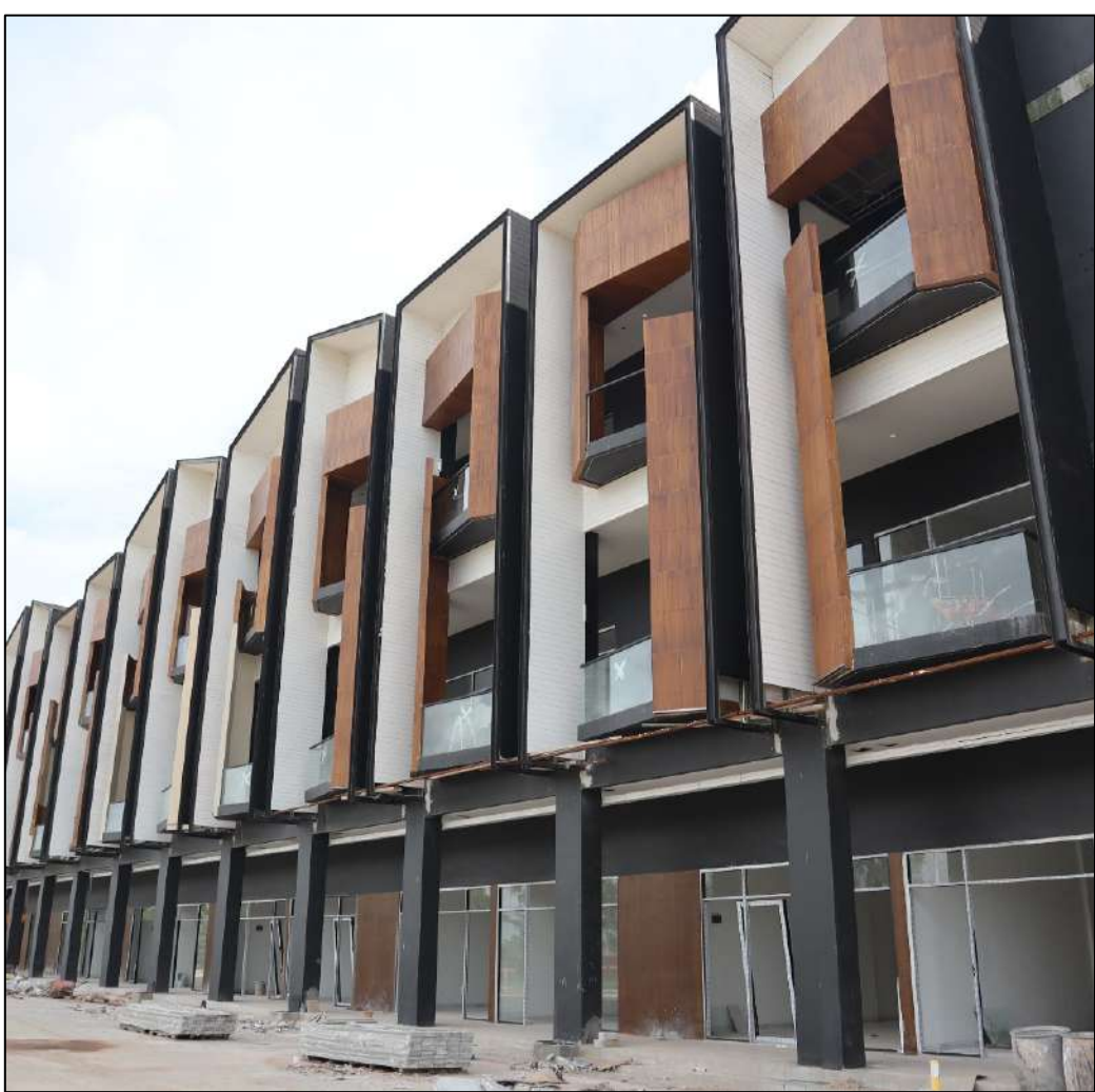
3 CEILING FRAME WORK PAUL LANE (SHOPHOUSE)
