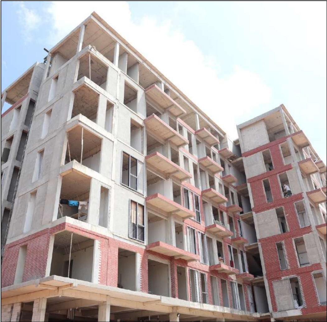
2 MANSORY, PLASTERING WORK (CONDOVILLA)
