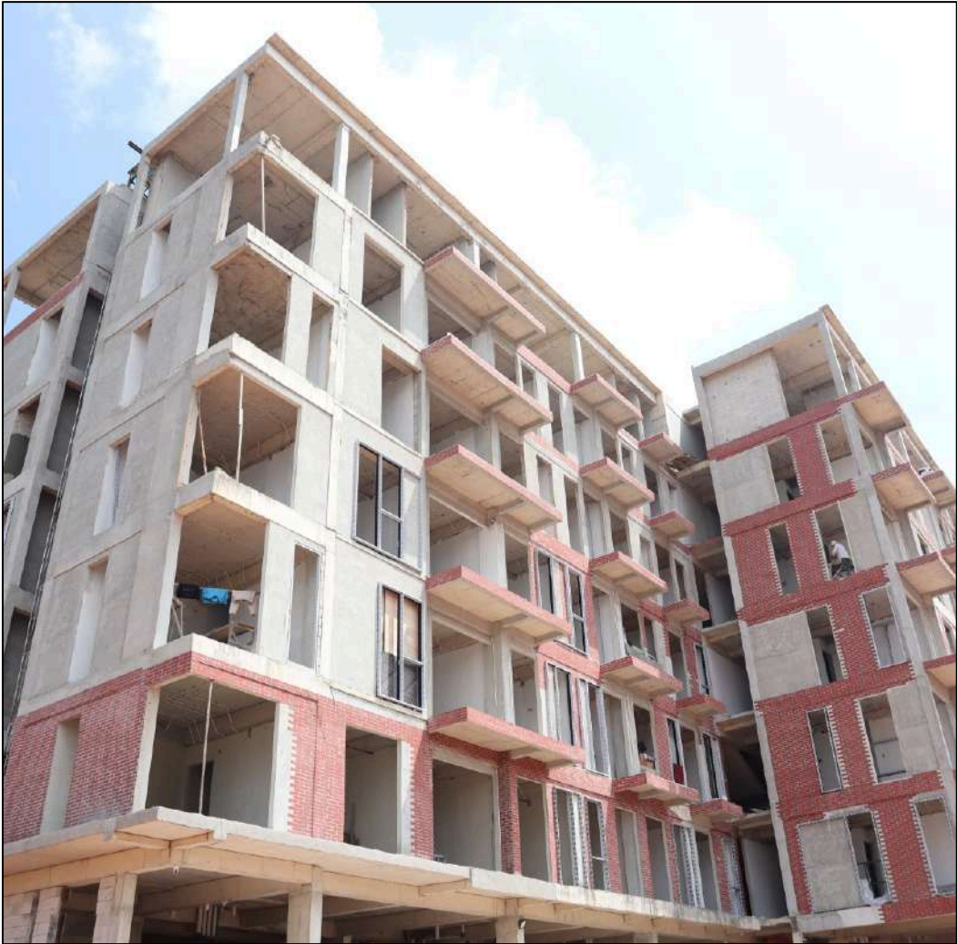
2 MANSORY, PLASTERING WORK (CONDOVILLA)
