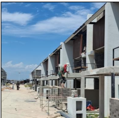
Construction Glenn The Hive (Landed House)
