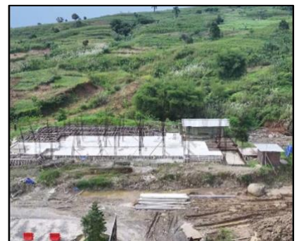
Construction Club House Cluster I: The Leroy
