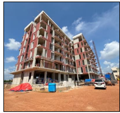
Construction of Condovilla
