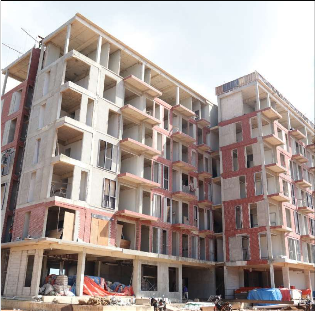
2 MANSORY, PLASTERING WORK (CONDOVILLA)
