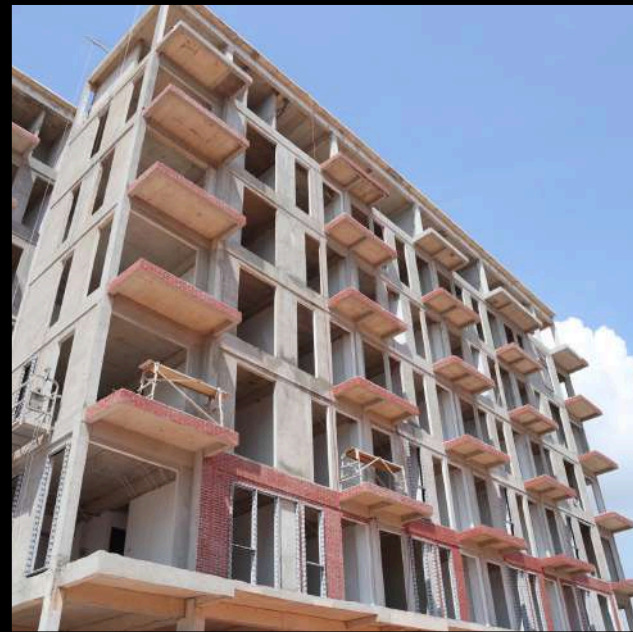
2 CONSTRUCTION OF PAUL & PRIVE (CONDOVILLA)
