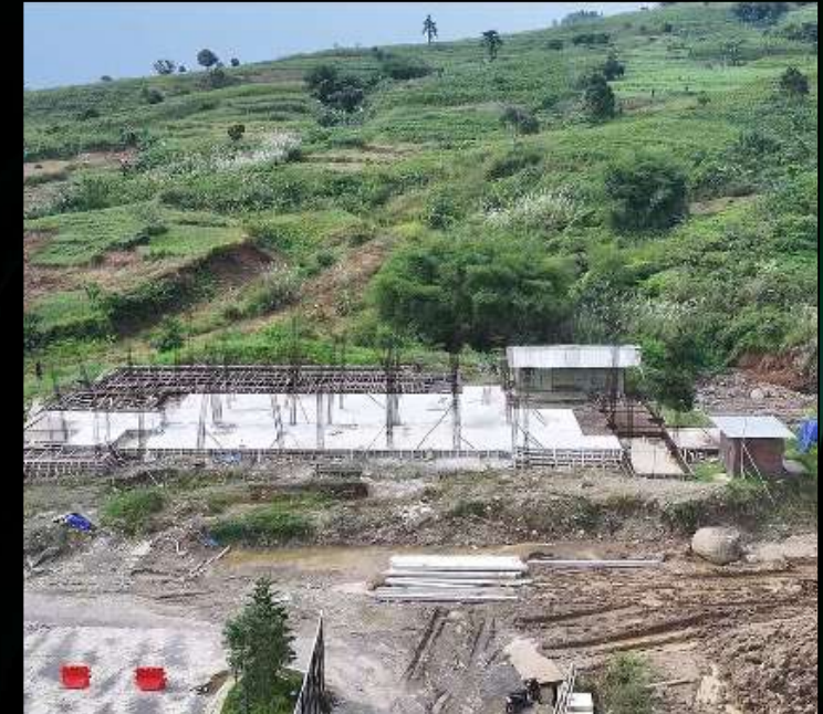
6 CONSTRUCTION OF CLUBHOUSE THE LEROY (CLUSTER I)
