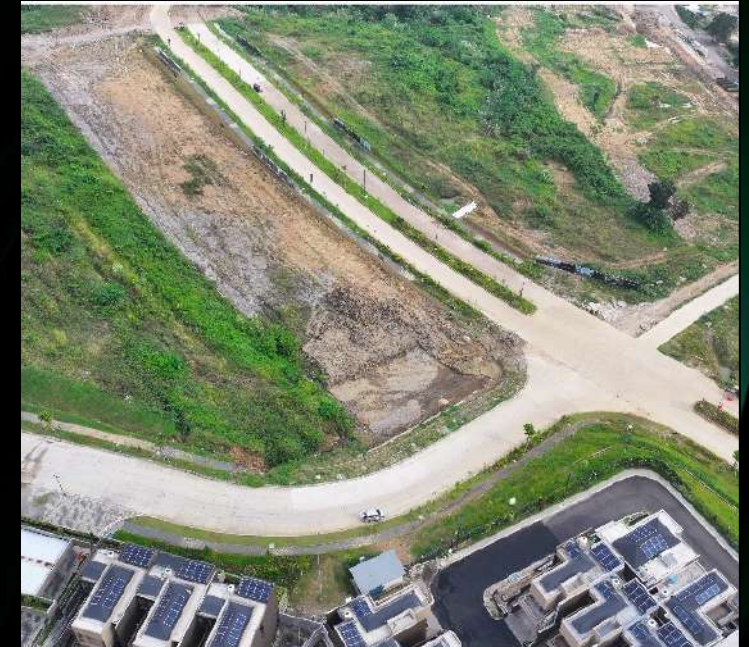
3 COMPLETION OF ROW 30 PHASE 2 (ROAD ACCESS TO BRIDGE 2 AND 3)
