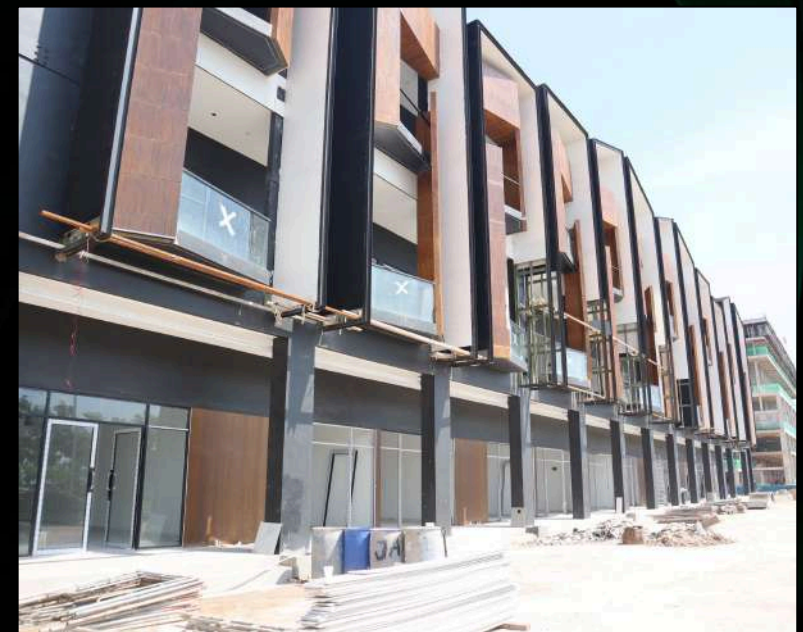
3 CONSTRUCTION OF PAUL LANE (SHOPHOUSE)
