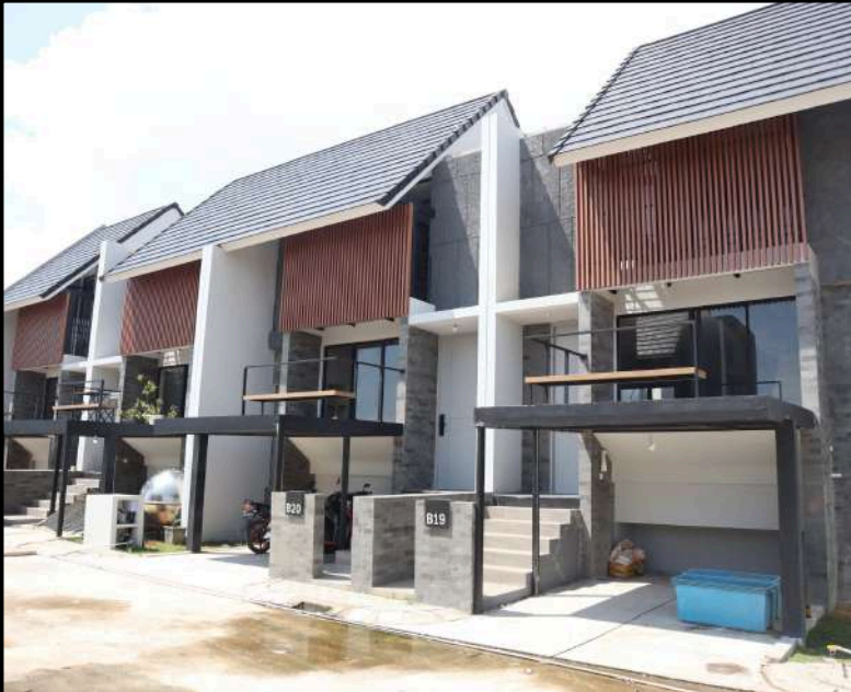
1 CONSTRUCTION OF GLENN THE HIVE (LANDED HOUSE)
