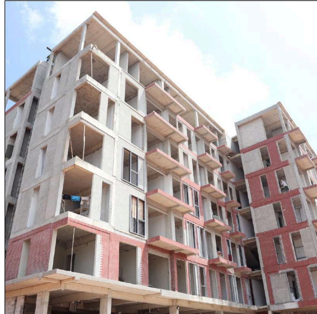
2 MANSORY, PLASTERING WORK (CONDOVILLA)
