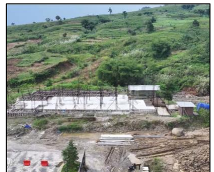
Construction Club House Cluster I: The Leroy
