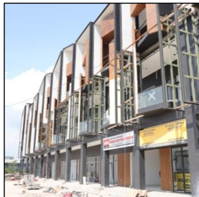
Construction of Shophouses
