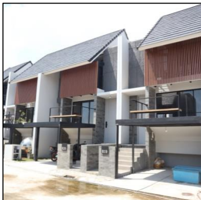
Construction Glenn The Hive (Landed House)
