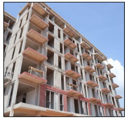
Construction of Condovilla
