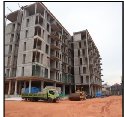
Construction of Condovilla
