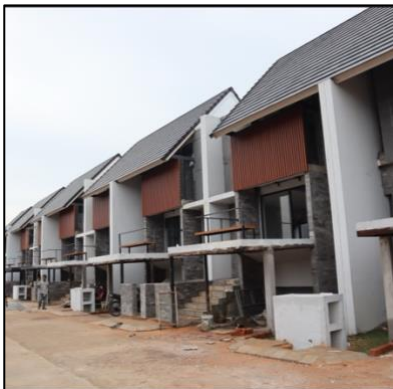
Construction Glenn The Hive (Landed House)
