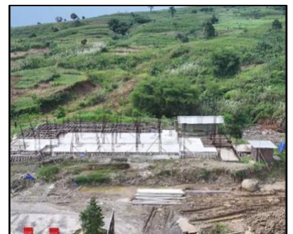
Construction Club House Cluster I: The Leroy
