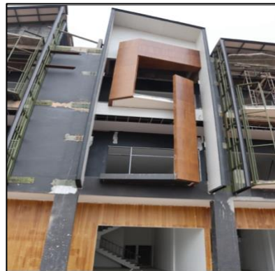
Construction of Shophouses
