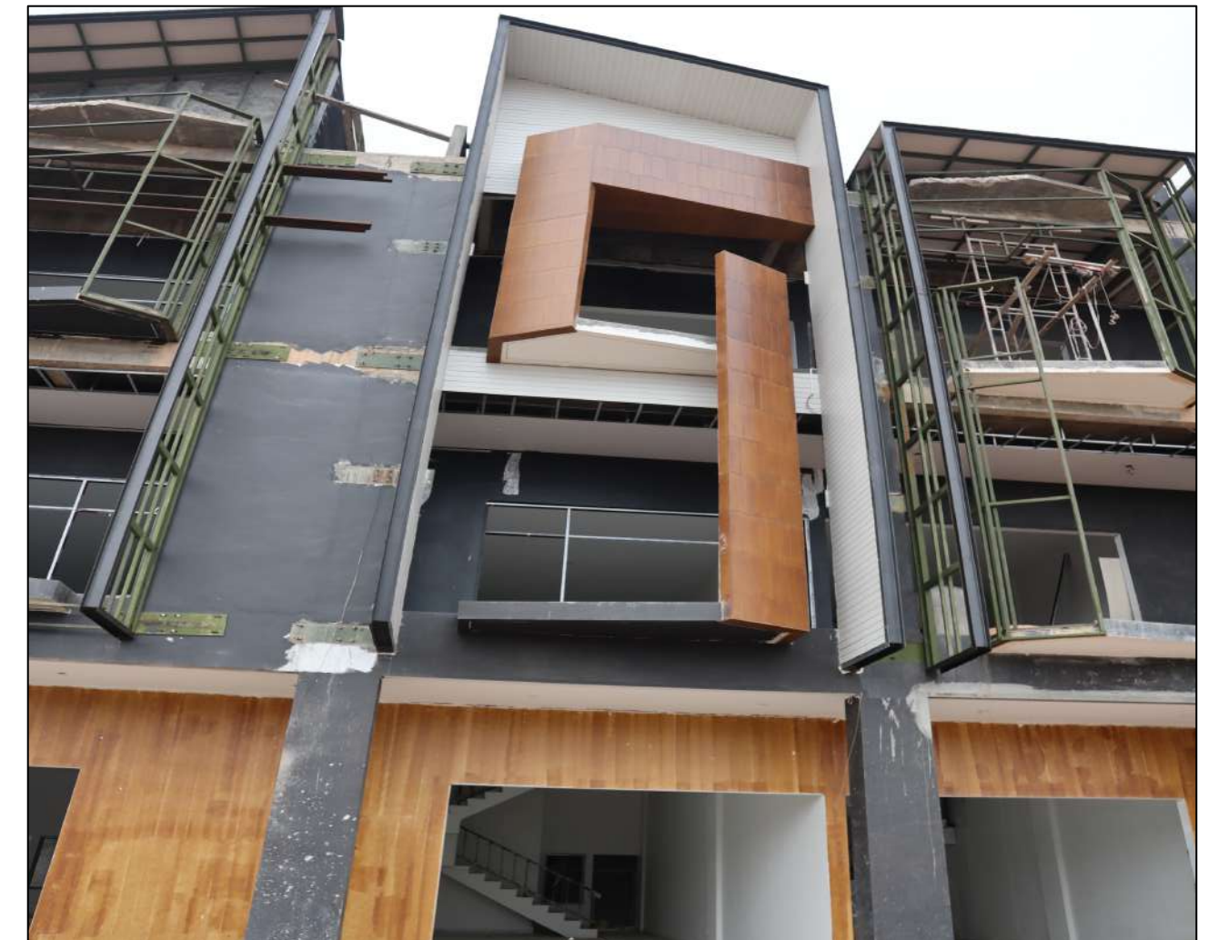
3 CEILING FRAME WORK PAUL LANE (SHOPHOUSE)
