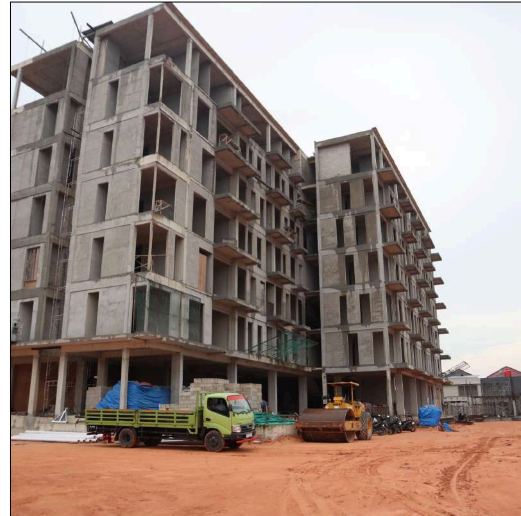
2 MANSORY, PLASTERING WORK (CONDOVILLA)
