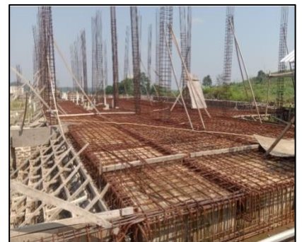
Construction Club House Cluster I: The Leroy
