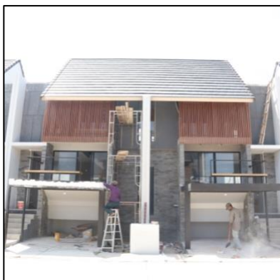
Construction Glenn The Hive (Landed House)
