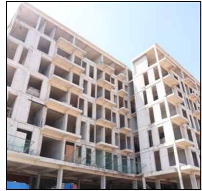
Construction of Condovilla
