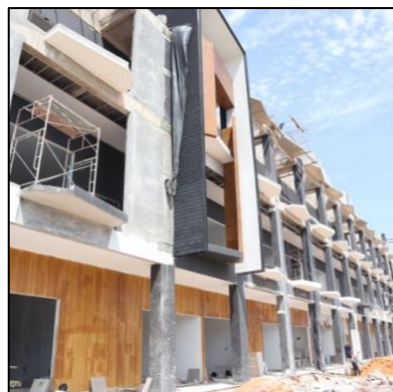
Construction of Shophouses
