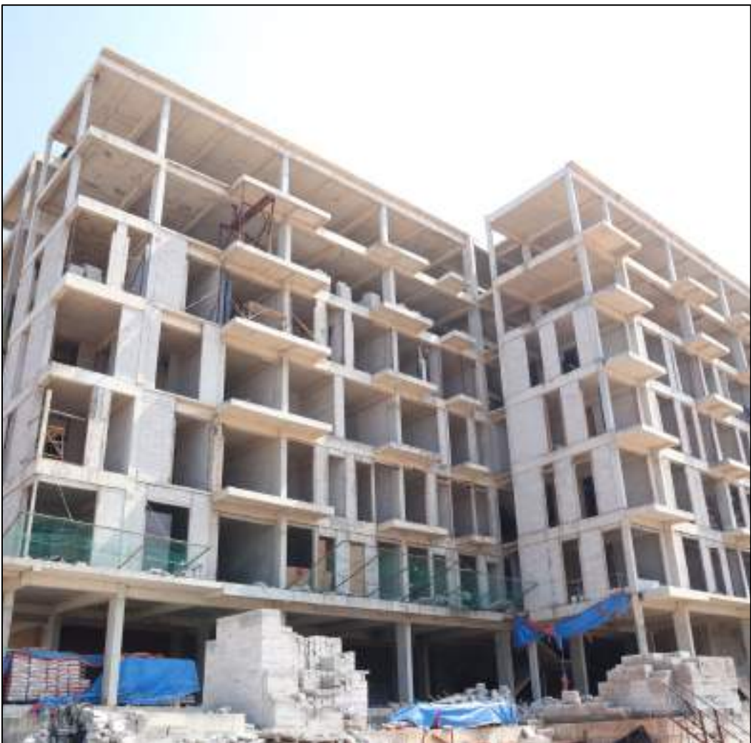
2 MANSORY, PLASTERING WORK (CONDOVILLA)
