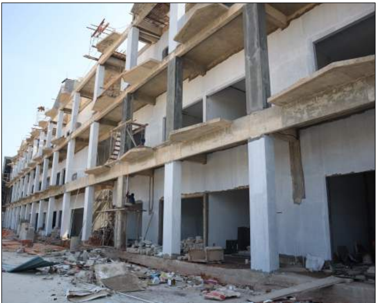
3 CEILING FRAME WORK PAUL LANE (SHOPHOUSE)
