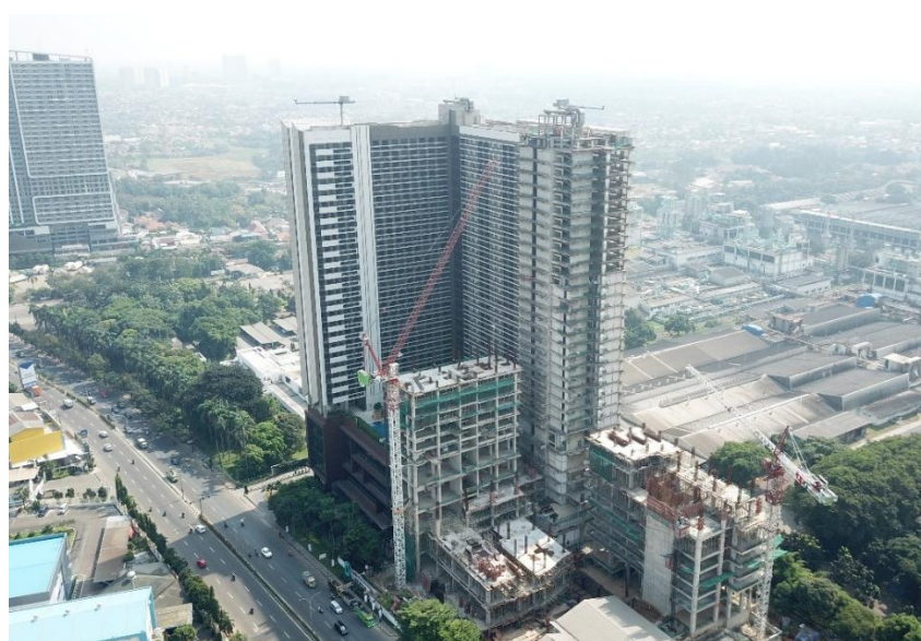
Photo: Construction progress of The Scott, Collins Boulevard, Tangerang
