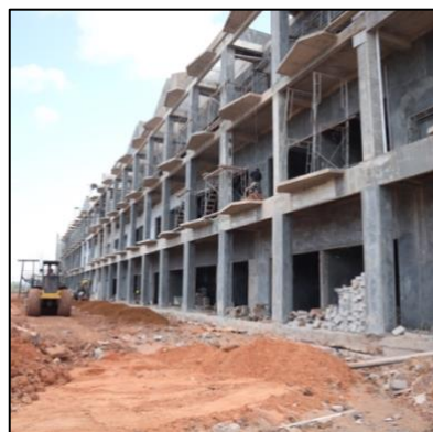
Construction of Shophouses
