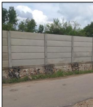
Fence Panel Installation Phase 4
