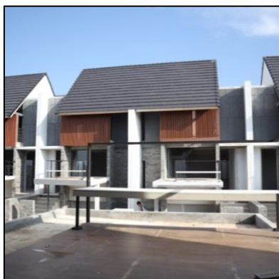
Construction Glenn The Hive (Landed House)
