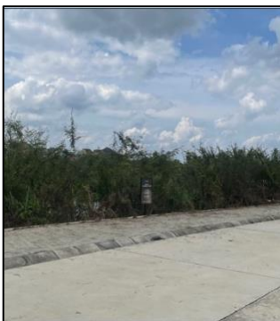
Pavement Work of ROW 20 Phase 1
