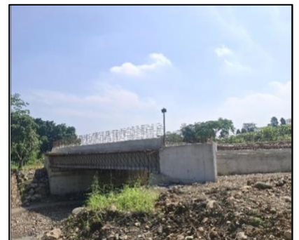
Completion of Superstructure Bridge 3
