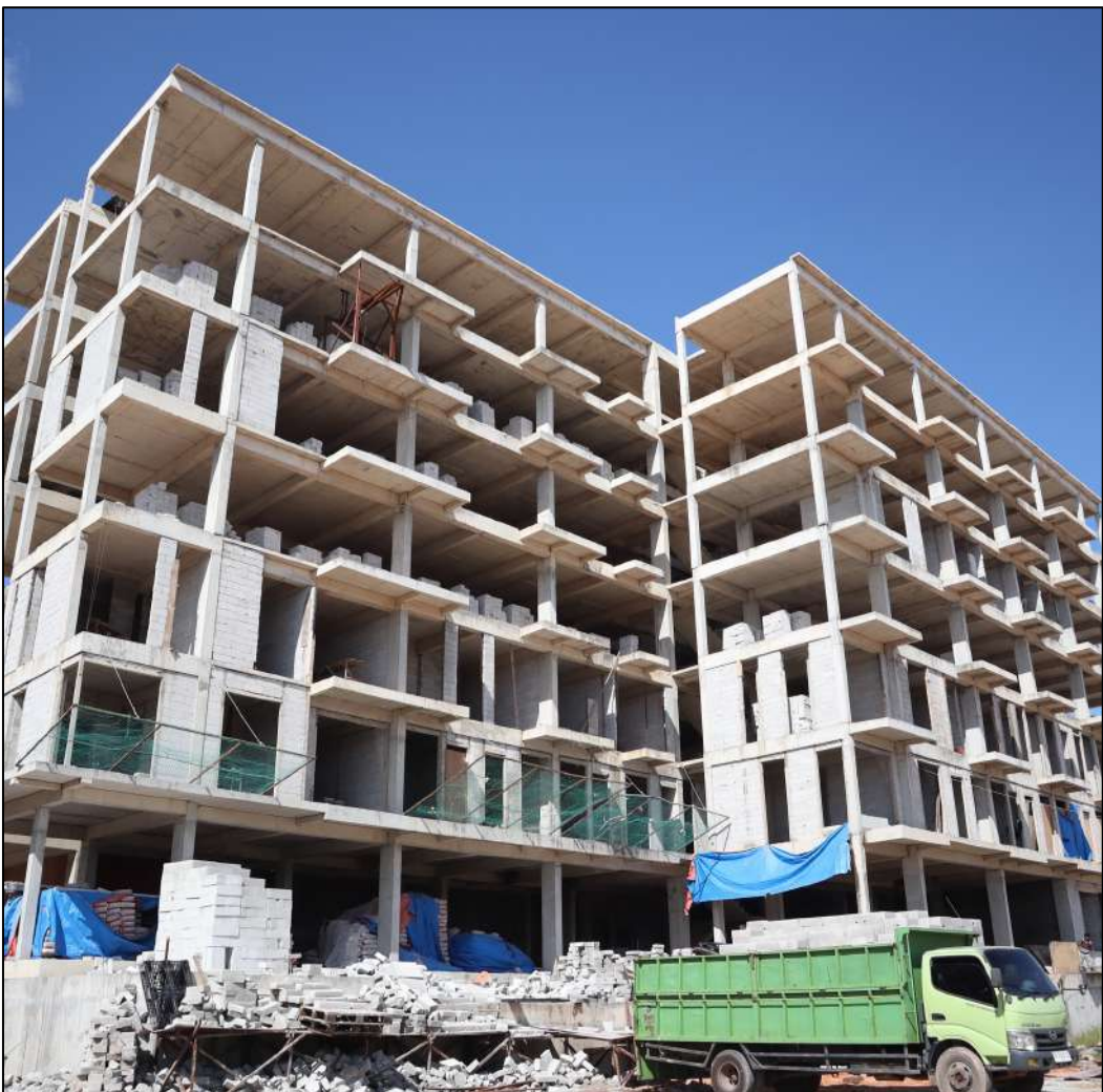
2 MANSORY, PLASTERING WORK (CONDOVILLA)
