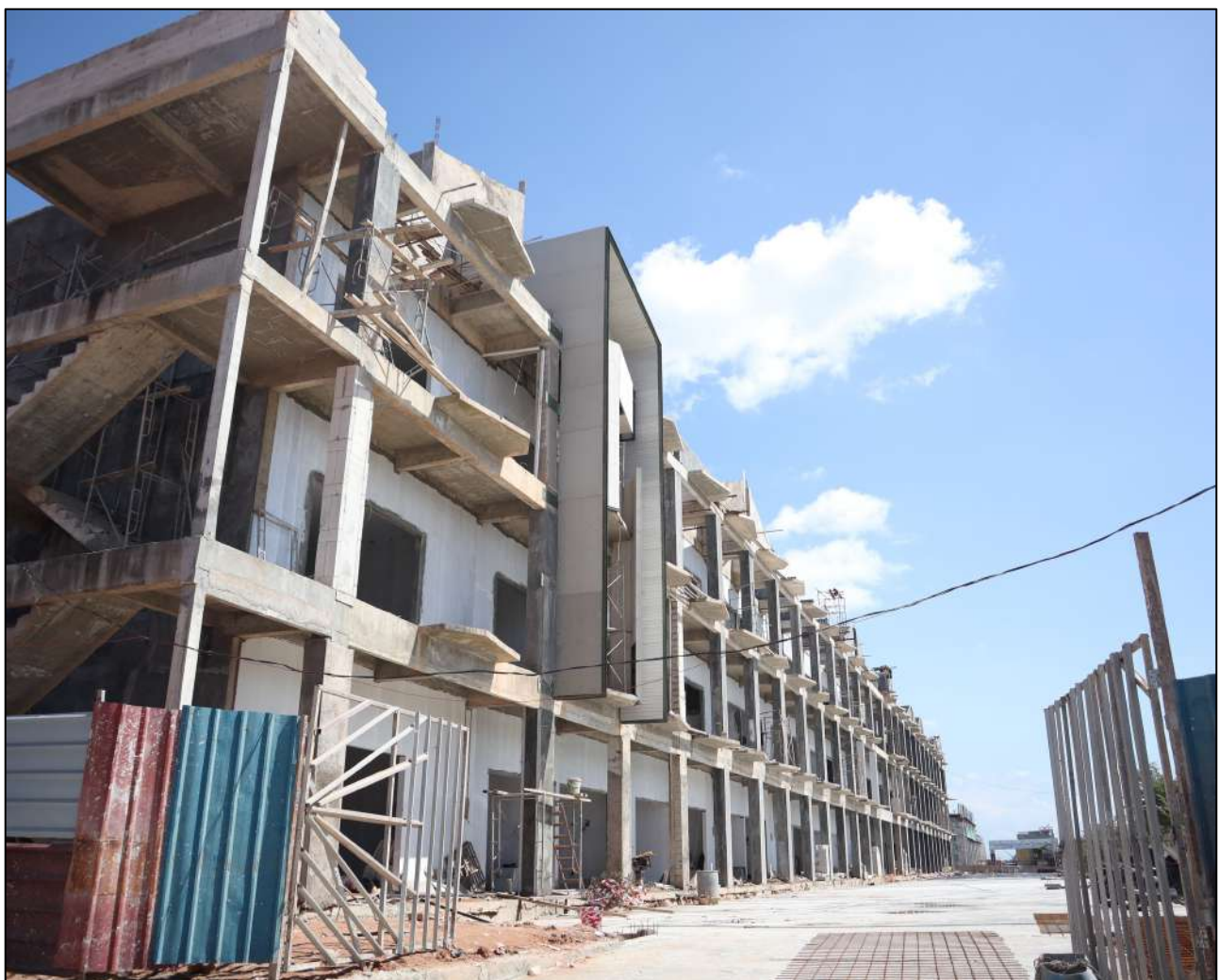
3 CEILING FRAME WORK PAUL LANE (SHOPHOUSE)
