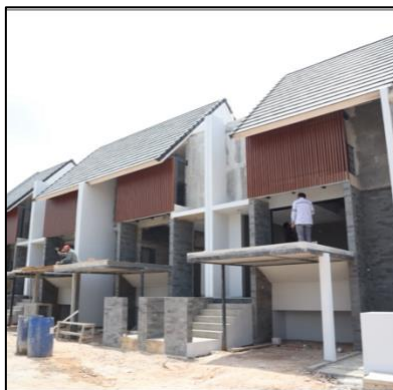
Construction Glenn The Hive (Landed House)
