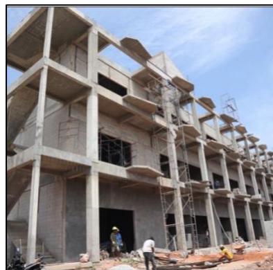
Construction of Shophouses
