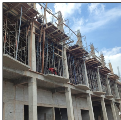
Construction of Shophouses
