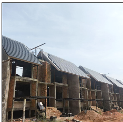
Construction Glenn The Hive (Landed House)
