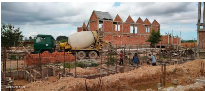
Residential Glenn the Hive Construction
