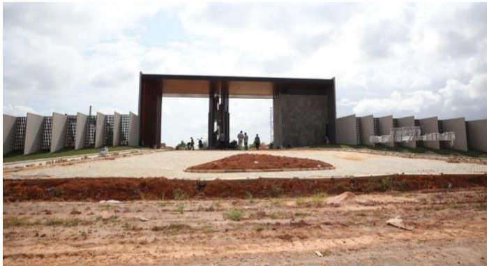
Main Gate Glenn The Hive Construction
