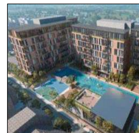
Persiapan Proyek Marc's Boulevard
