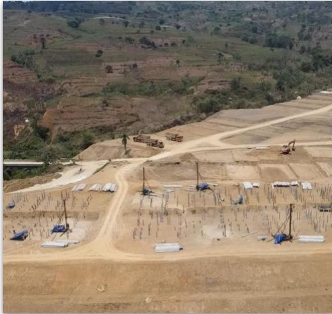
Figure IV. Construction of piles for The Leroy Cluster I as of October 31, 2023
