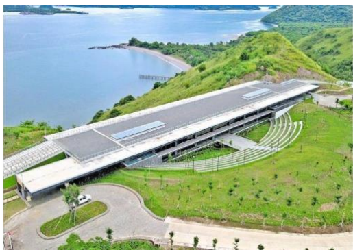
Figure VIII. Path Walk construction progress as of October 31, 2023
