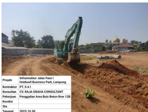
Figure II. Road Infrastructure Development
