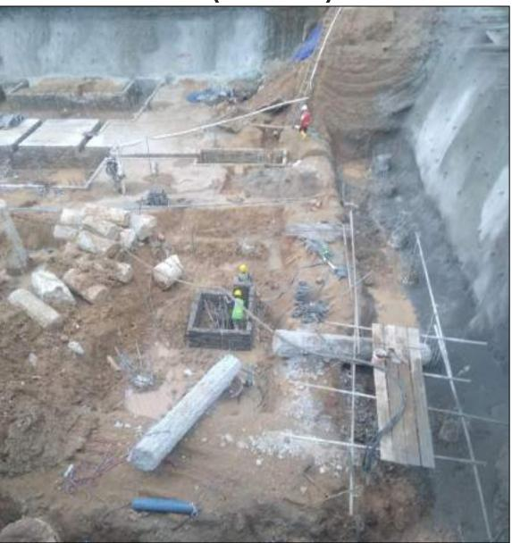
INSTALLATION OF EXCAVATION SLOPE REINFORCEMENT (TOWER II)
