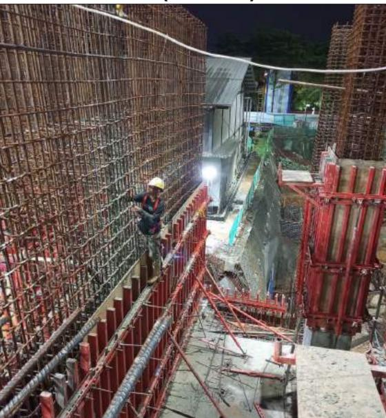
INSTALLATION OF EXCAVATION SLOPE REINFORCEMENT (TOWER II)
