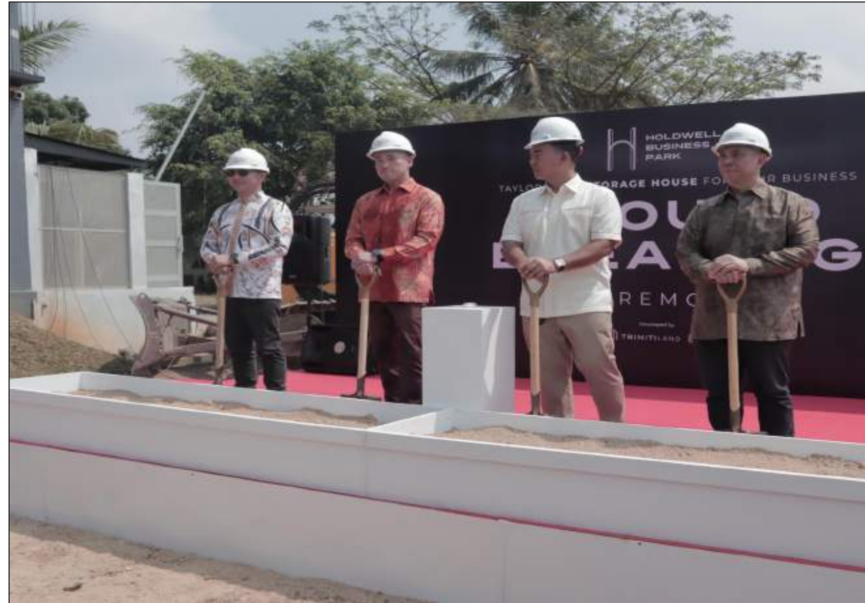
Ground Breaking Holdwell Business Park
