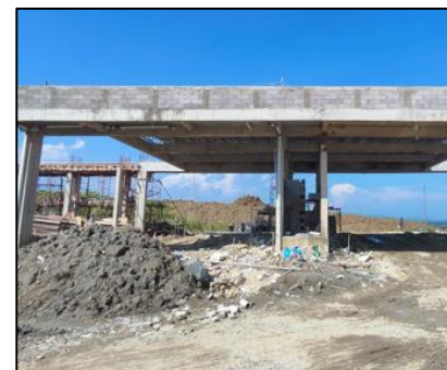
Gate Structure Cluster I
