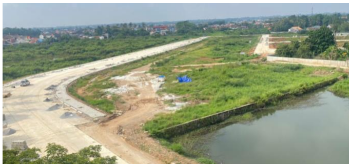
Infrastructure Phase I
