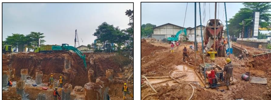
Construction Progress of Collins Tower II
