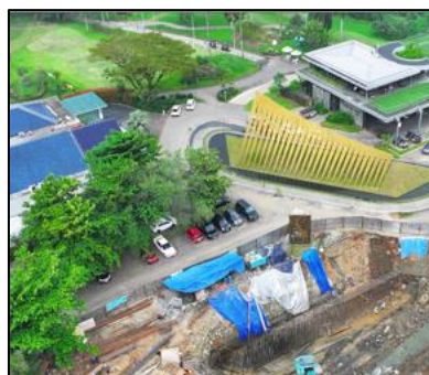
Bridge 1 Main Gate
